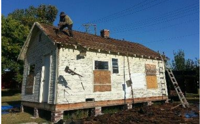
Work on the roof is now underway.
