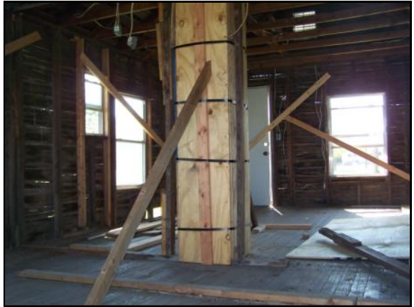
The interior of the schoolhouse is braced for the move to the museum
